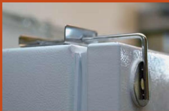
Research equipment is seismically restrained in earthquake-prone areas.
